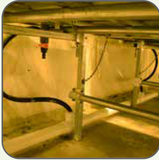
Figure 6: Example of piped drainage from trays
